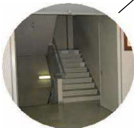
屋内階段と防火戸
